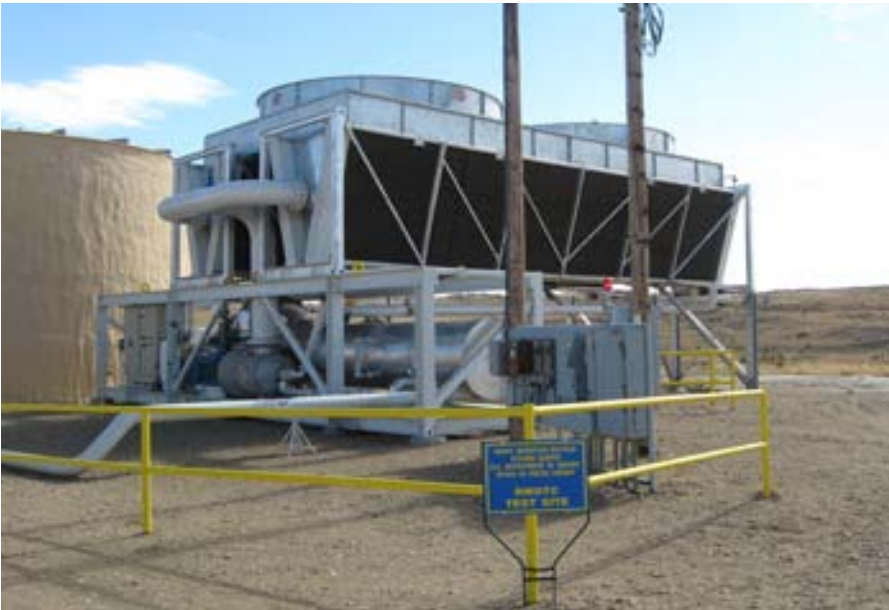
Source: DOE – Rocky Mountain Testing Center
