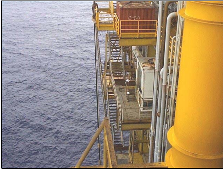
Fig. 15 Offshore Installation of Process Centrifuge
