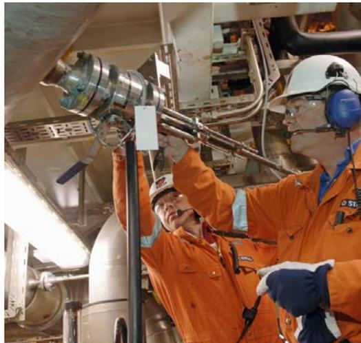
Figure 3: Inspection of inline sensor probe (Photo: StatoilHydro).
