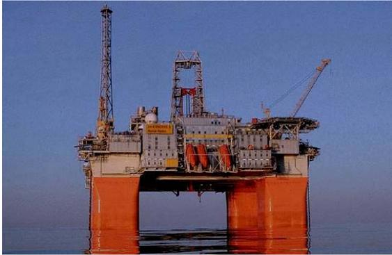
Located in the Tampen area of the Norwegian North Sea, the Snorre field has been producing oil and gas since August 1992. The Snorre development embraces two platforms, A and B. The Snorre B platform, a submersible PDQ floater came on stream in June 2001. Oil from Snorre B is piped to Statfjord B for storage and export. The gas can be injected back into the reservoir, or (partly) transported by pipeline via Snorre A to the Statpipe/Norpipe system.
